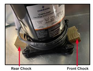
Figure 5. Compressor Chock Removal
